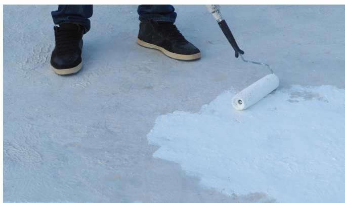
A roof being coated with Topps Seal.
