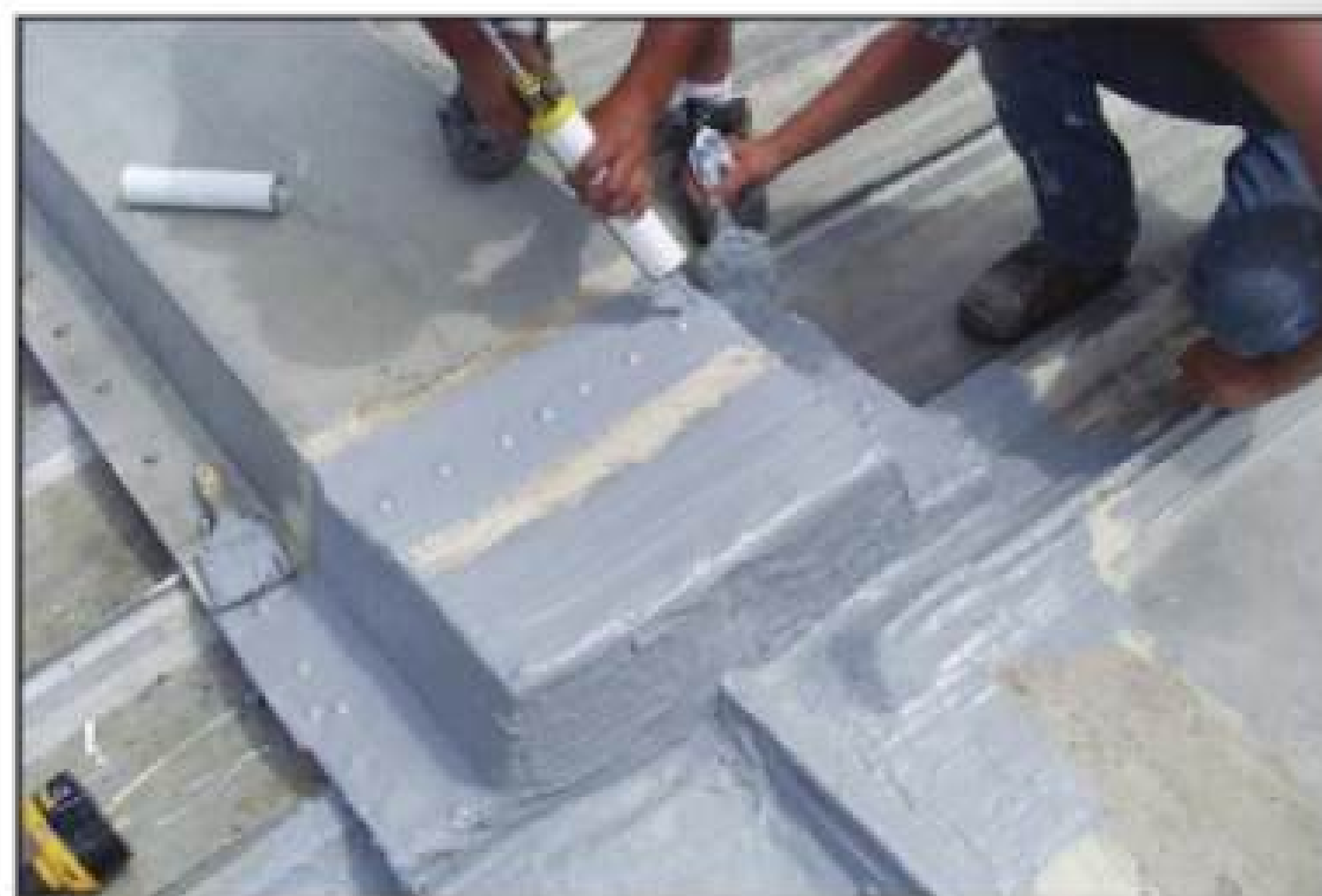
It's easy to apply Polyprene® from available caulk tubes precisely where you need it.
