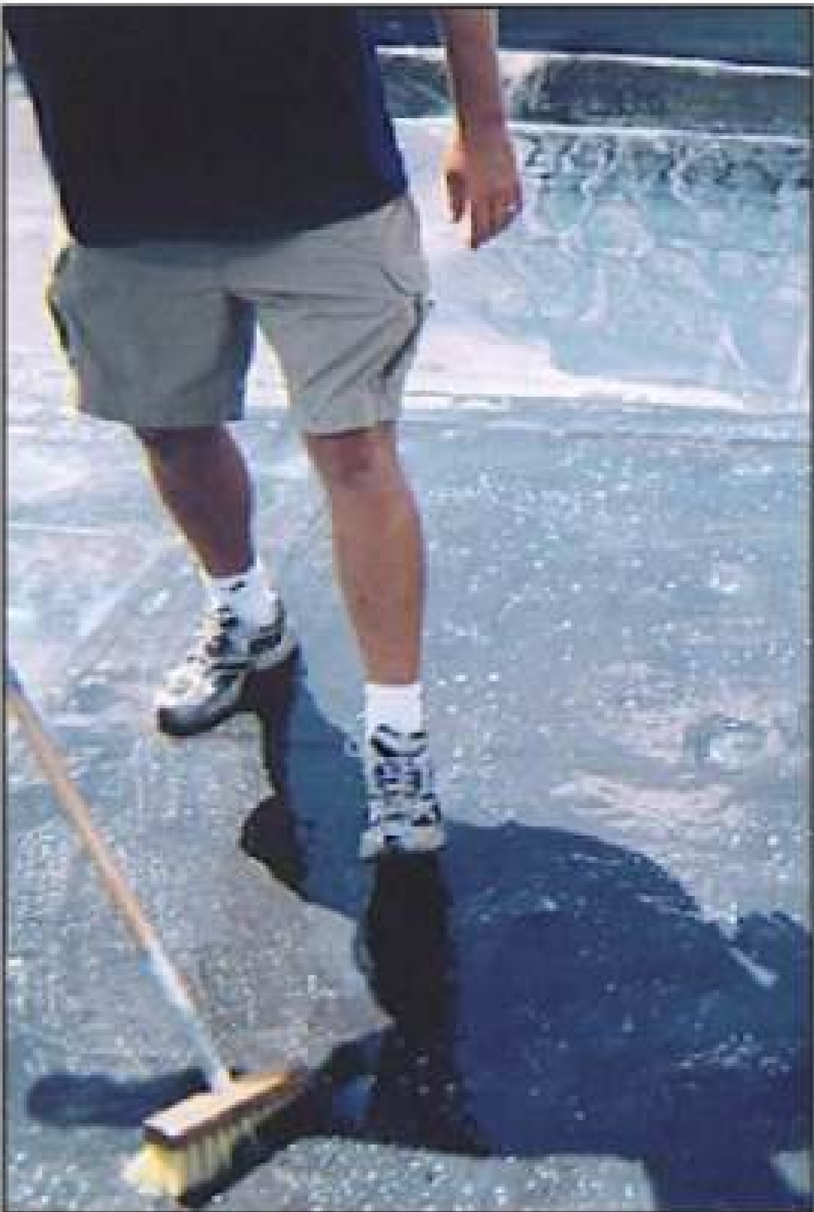
BUR roof being cleaned with MultiUse Cleaner
