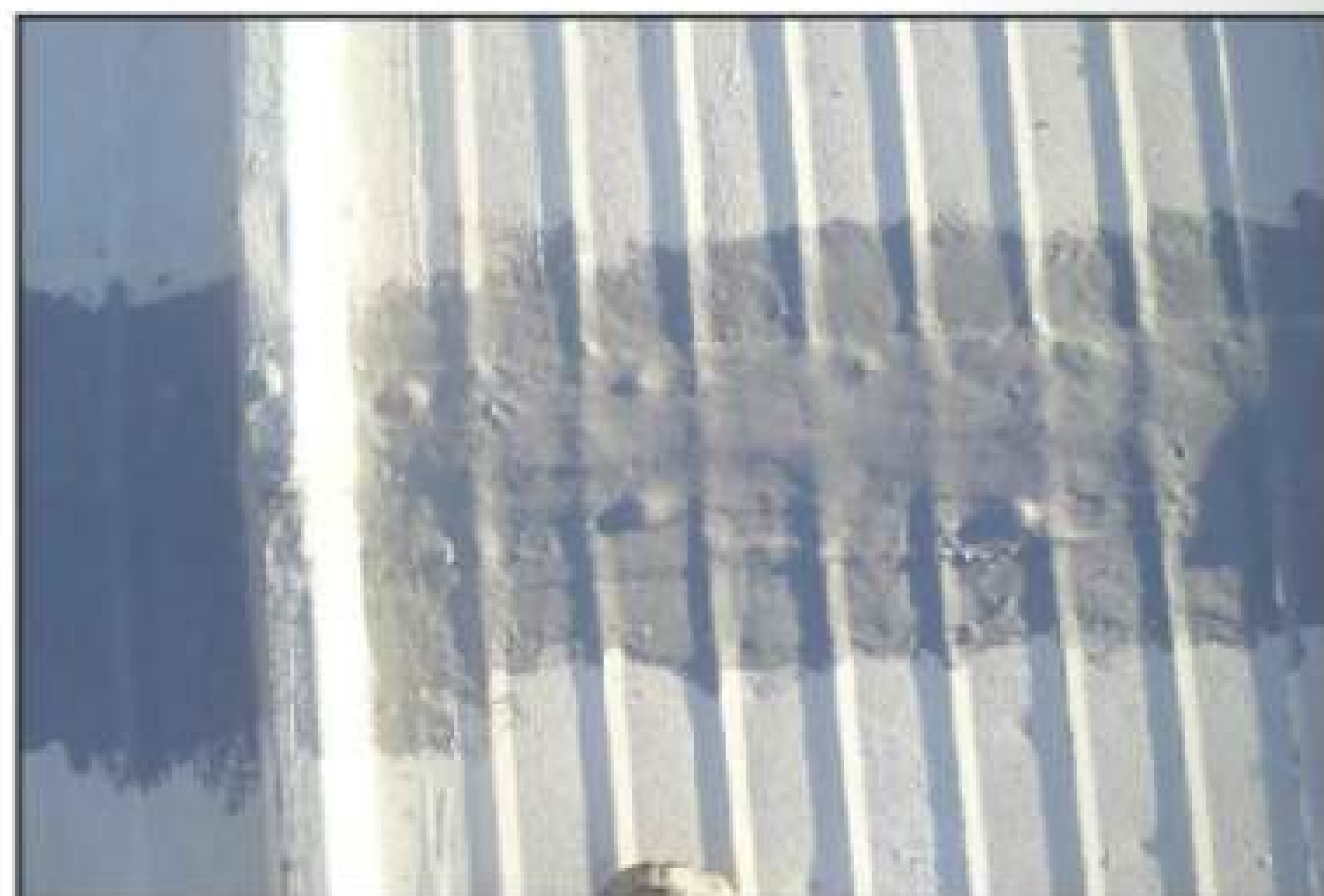
PolyCore™ is embedded between layers of Polyprene® to strengthen a repair.
