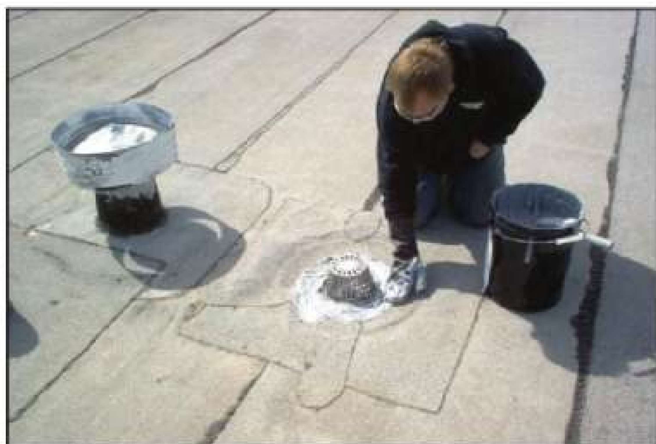
Polyprene®, applied around drain by hand, easily fills the voids that let in water.
