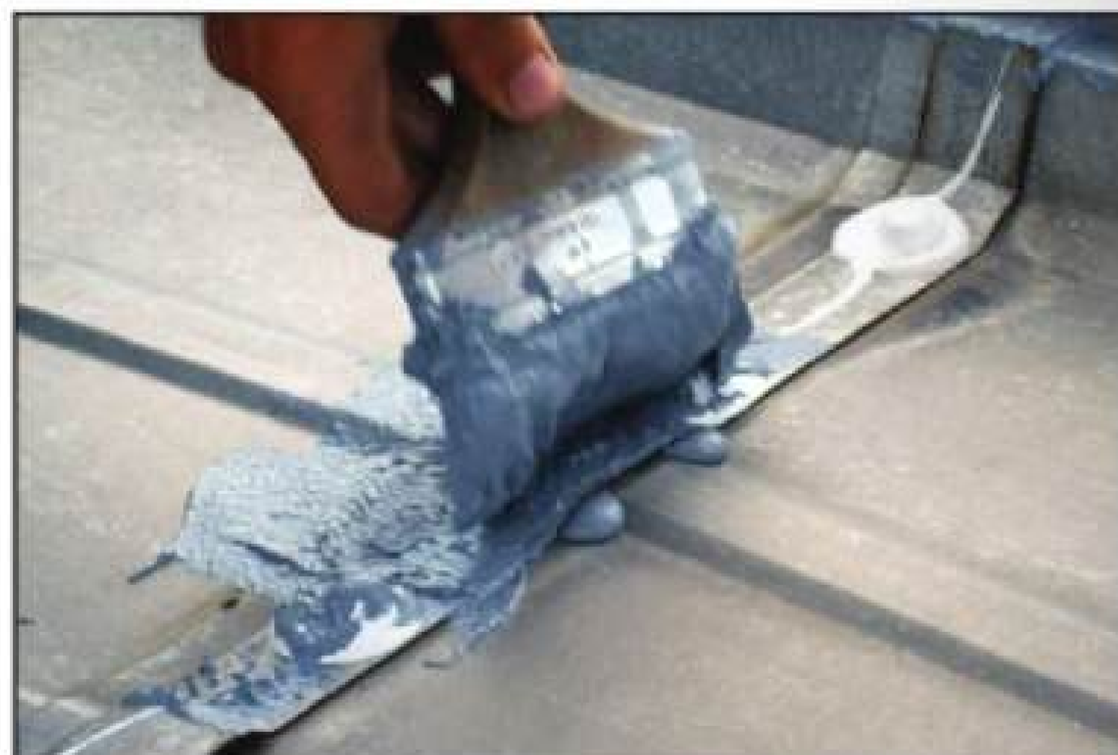
Polyprene® is brushed over any seam, sealing it instantly. Note beads of Polyprene applied under metal seam (below brush).
